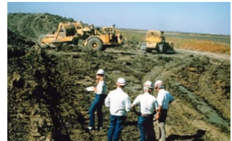
Colusa Basin Levee
