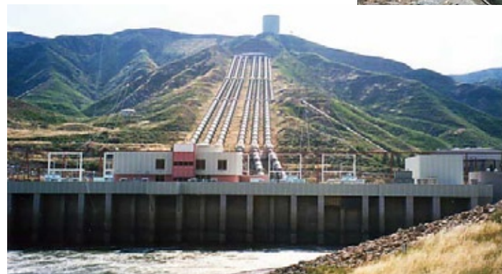
Castaic Power Plant
