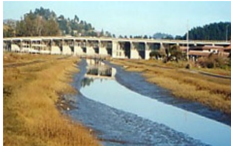
Richardson Bay Bridge
